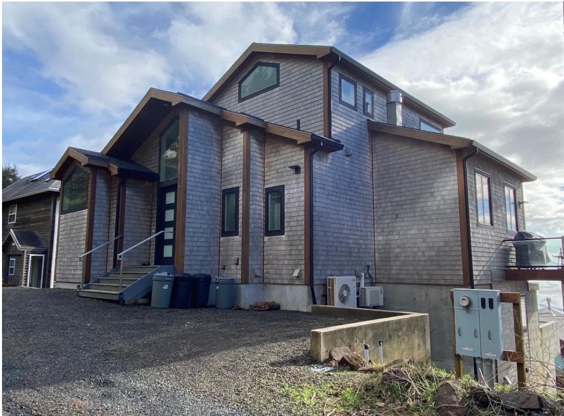
Exhibit 1A: Uphill side
