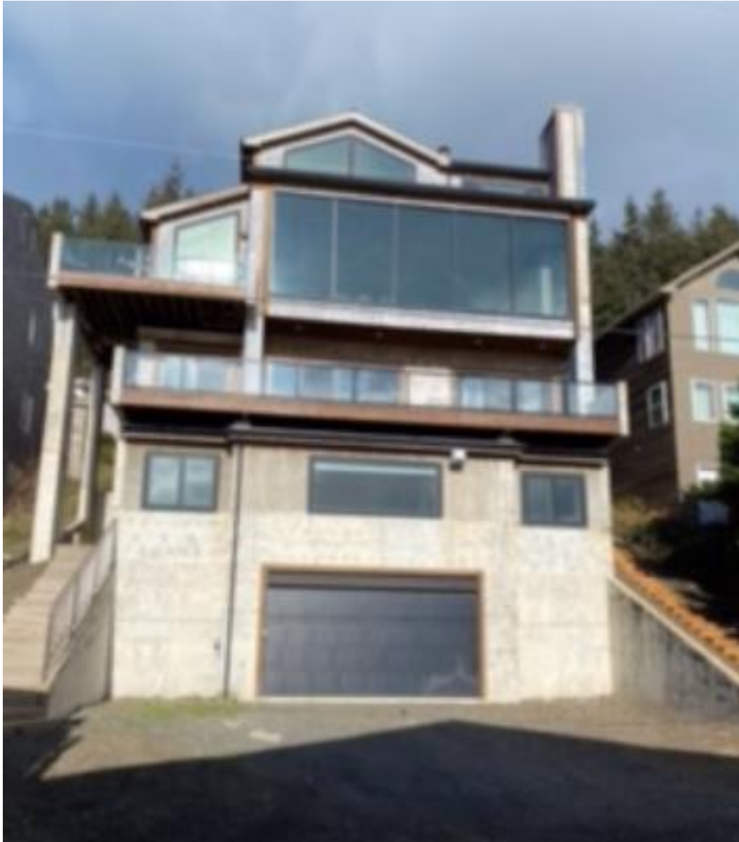
Exhibit 1B: Downhill side of the same house
